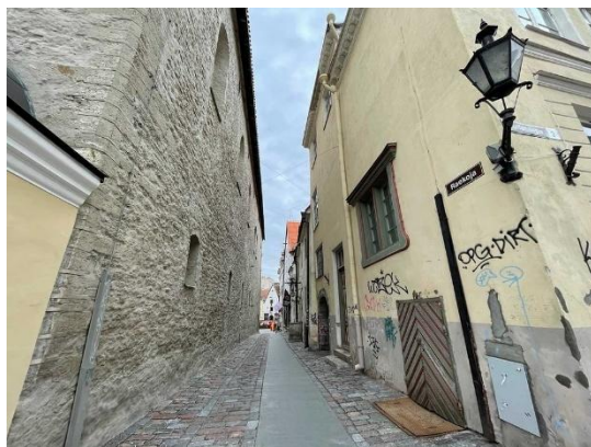
Fig. 2.9 — Localised inserts of smooth tiles or strips that make key points (entrances, bus stops, crossings) more accessible without altering the entire area. A street in Tallinn, Estonia (WheelchairTravel.org, 2023)
