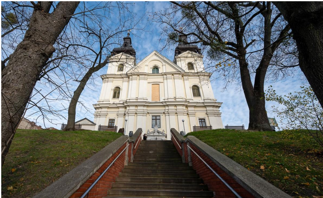
Fig. 2.35 — Stairs leading to the Church of St Michael the Archangel, which create a barrier for people with mobility impairments, Lviv (Your City, 2023)
