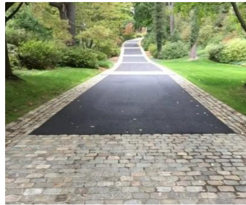
Fig. 2.8 — Part of the surface covered with a modern layer (asphalt) to create smooth routes (Stone Curators, 2025)
