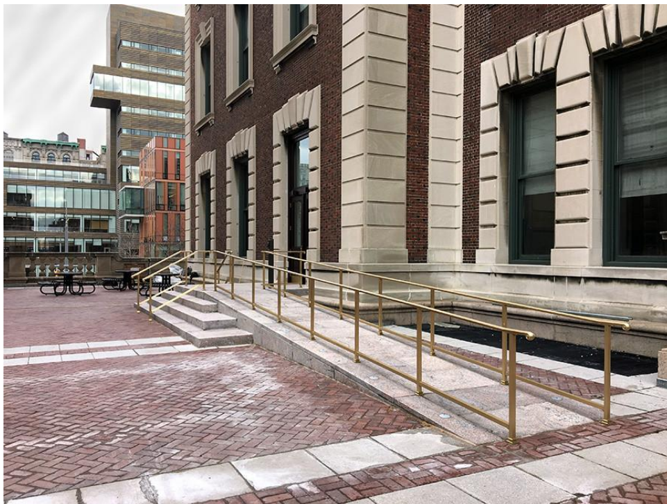
Fig. 2.11 — Example of a ramp leading to the entrance of Columbia University's Morningside campus (Columbia News, 2019)
