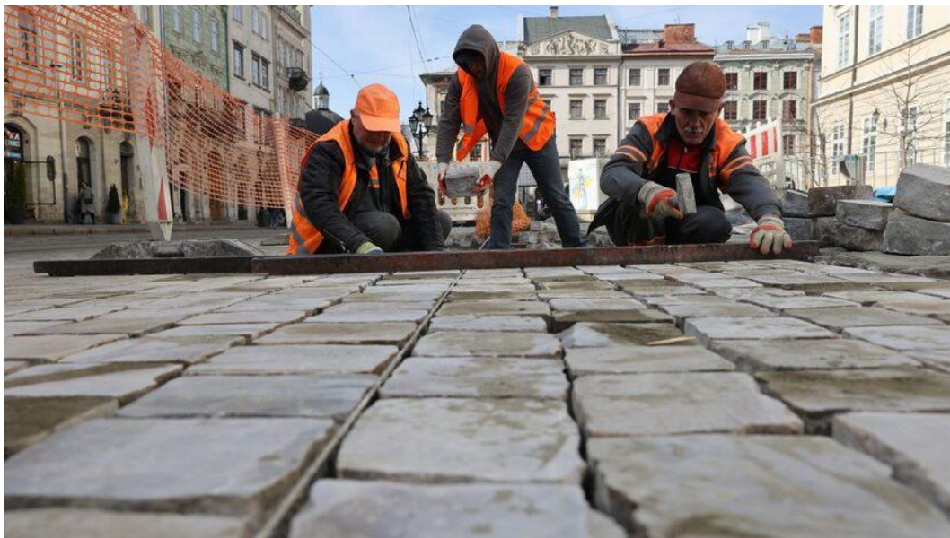
Fig. 2.51 — Lviv has adopted an interesting solution from several European cities for improving accessibility on cobbled streets and squares — accessibility paths. The cobblestones are removed and ground down to a smooth, level surface without any unevenness. The thickness of the paving remains the same, averaging 17 centimetres, but its surface becomes level: this makes it easier for people in wheelchairs and with pushchairs to get through (Lviv City Council, 2025).
