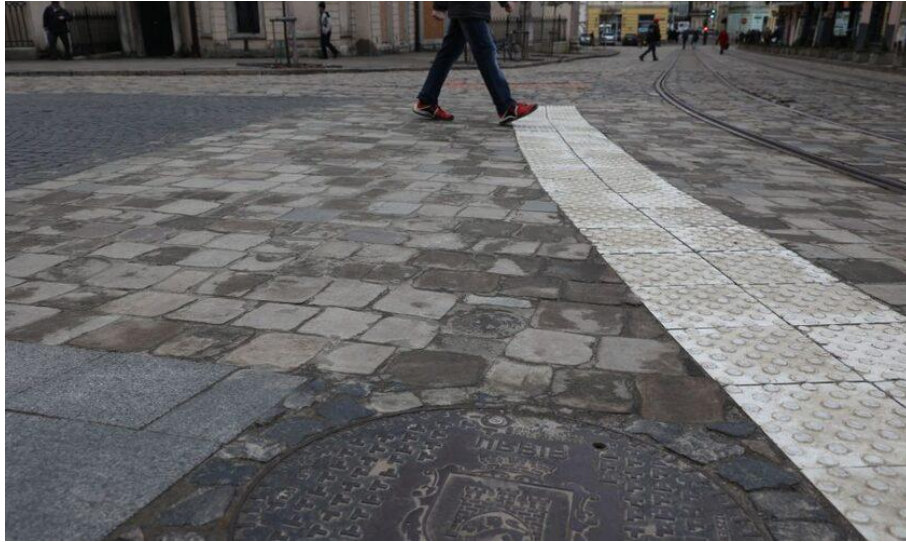
Fig. 2.48 — Improved pavement and installed tactile strips on Rynok Square in Lviv (Roman Baluk)
