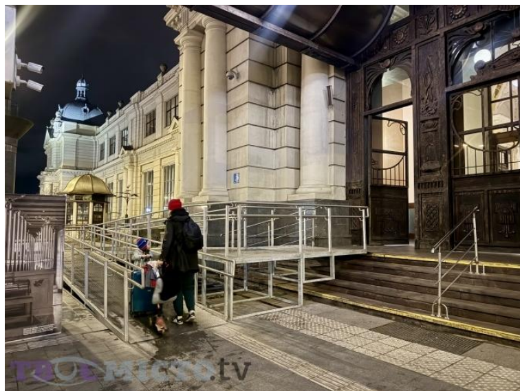
Fig. 2.47 — Ramp at the main entrance to Lviv railway station — an example of a temporary/modular structure that makes the historic building more accessible without significant alteration to the façade itself (Your City, 2025)
