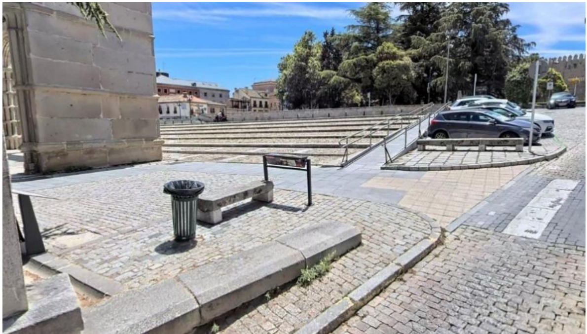
Fig. 2.44 — Ramp and information stands for people with disabilities at the entrance to the Basilica de San Vicente in Ávila, Spain (Apple Maps, n.d.)
