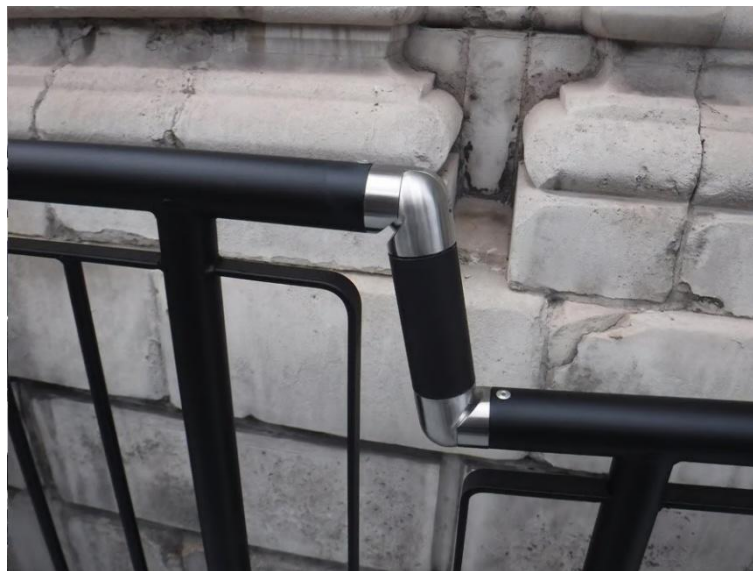
Fig. 2.23 — Handrails made from a material that is comfortable to use in cold weather (Rapid Ramp, 2019)
