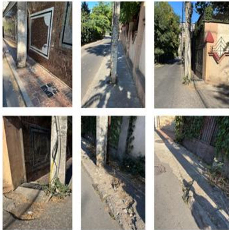
Fig. 14. The historic city of Odessa (Ukraine). Obstacles to movement: high kerbs, narrow pavements, obstacles in the form of trees, posts on pedestrian walkways, uneven or slippery surfaces. (Larysa Bridnia, 2025)
