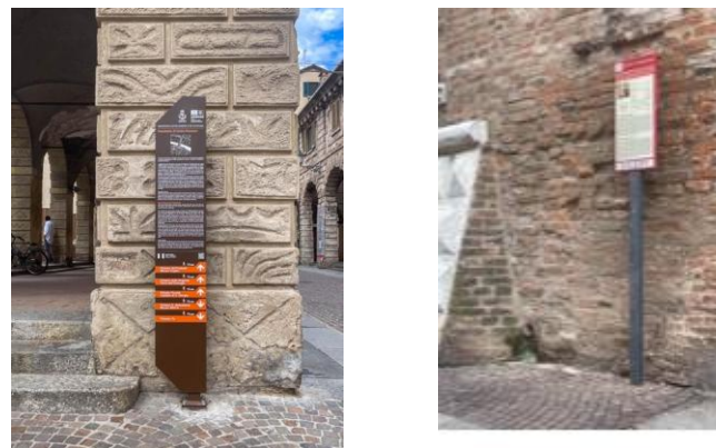
Figure 54 - 55. City of Mantua. Two examples of information panels in public space. In the image on the left, the excessive amount of text and the presence of non-relevant directional information make the panel inaccessible for people with cognitive disabilities and for blind or visually impaired users, due to the lack of appropriate graphic solutions and tactile information. In the image on the right, additionally, the graphic choices and the positioning of the panel hinder readability for several users, including wheelchair ones and children (Sebastiano Marconcini, 2025)
