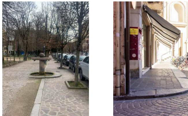
Figure 52 - 53. City of Mantua. In the image on the left, a fountain is located at the intersection between the sidewalk and the adjacent square. This element, along with the surrounding trees, obstructs the pedestrian path and represents a potential tripping hazard. In the image on the right, an example of a suspended obstacle - in this case, a mailbox that is not detectable by the white cane, posing a potential danger to visually impaired pedestrians (Francesca Paiola, 2025 e Sebastiano Marconcini, 2023)
