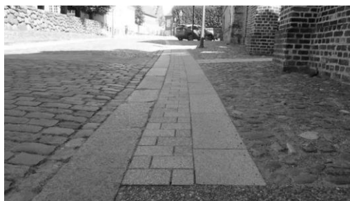
Figure 57. Viborg. Detail of the paving of a historical road, where it was designed a lane with features that allow a comfortable and safe use of the spaces for everyone (Source: https://realdania.dk/projekter/tilgaengelighed-historiske-bykerner )
