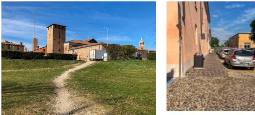
Figure 48 - 49. City of Mantua. The first image shows the connection path between the historic centre and the lake par of the city, where the transition occurs through an irregular ramp, of unsuitable materials and excessive slope. In the image on the right, a connecting ramp between the street and sidewalk is shown, with a slope greater than 10%, making it unsuitable for safe and accessible use (Sebastiano Marconcini, 2025)
